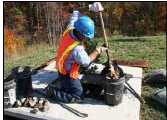
2. Removal of tree grate and erosion control stones
