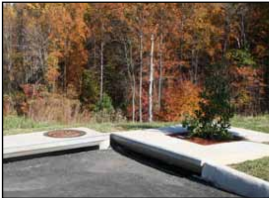
1. Inspection of Filterra and surrounding area
