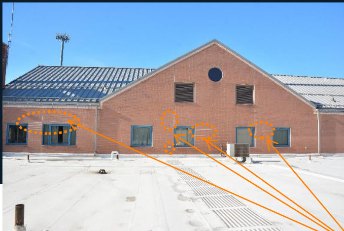
Example of improperly fastened counterflashings
