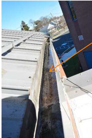
Example of water sitting in dead level gutter, no pitch to downspout outlets.
