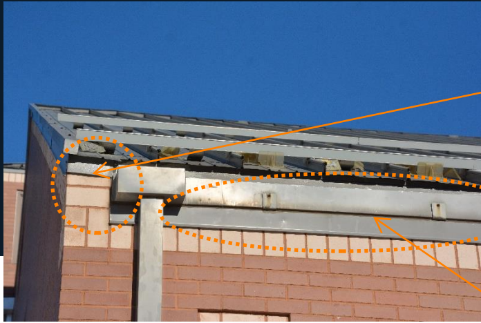
Example of gutter stopping short of the edge of the roof.
