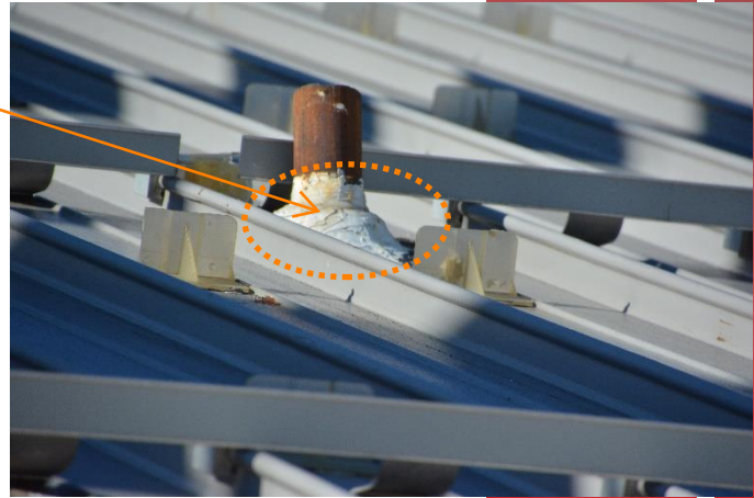
Example of stepped flashing with open sides.
