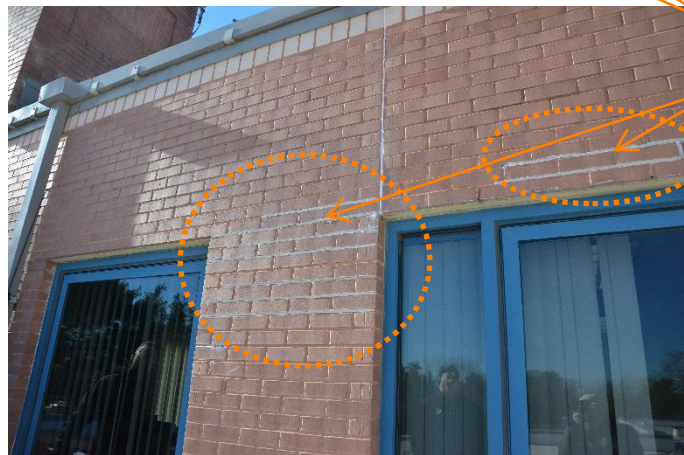
Examples of failing brick mortar and sealant joints.
