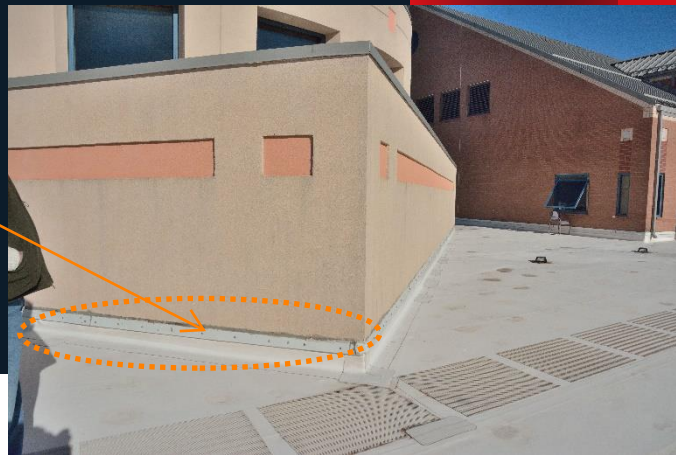
Examples of failing brick mortar and sealant joints.
