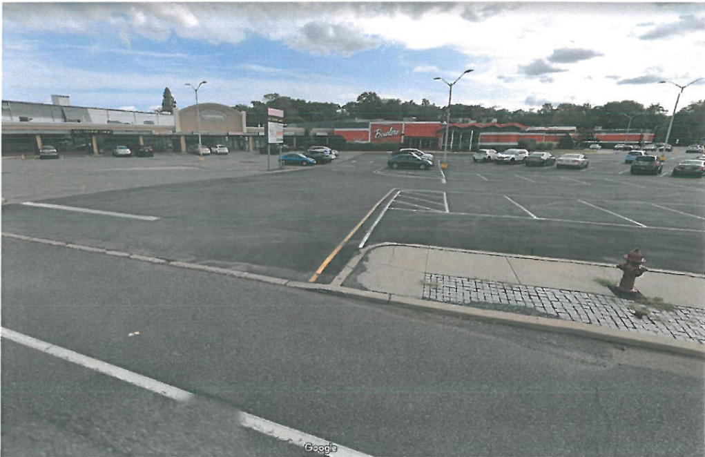
Figure 2: Subject property (Street view).
