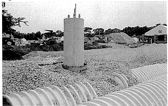
Figure 15 - Chamber bed placed around light post.
