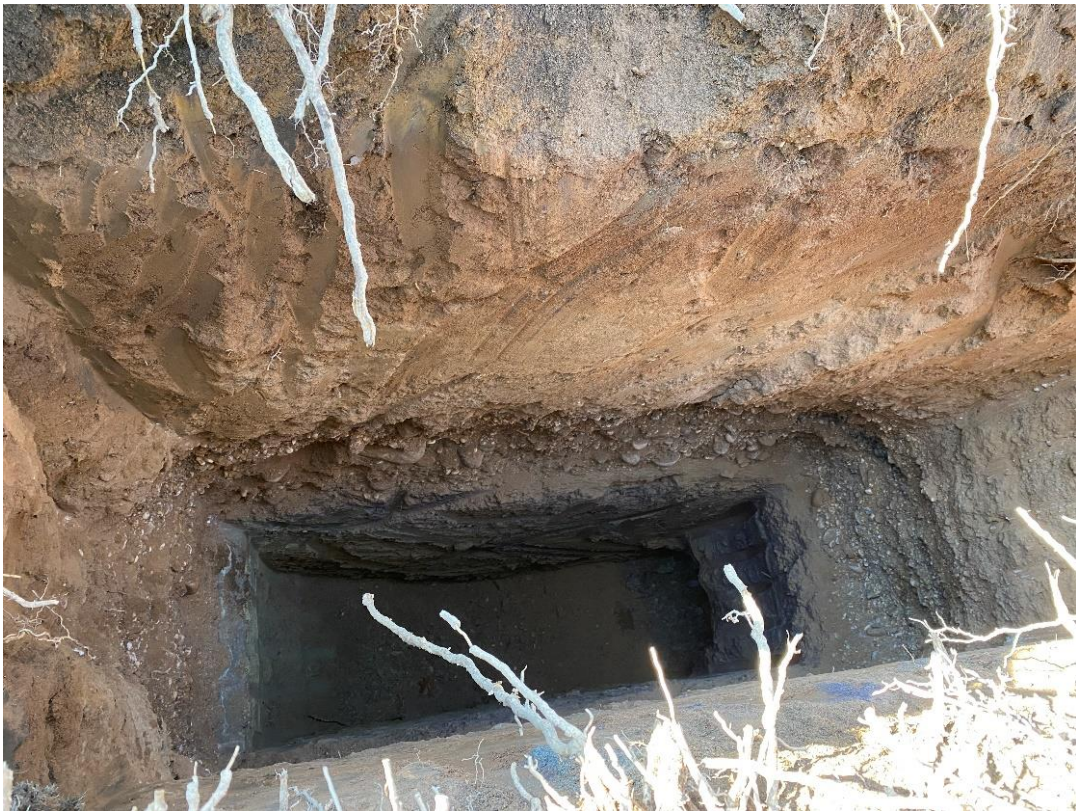
Photo 25: Profile of Test Pit TP-11.
