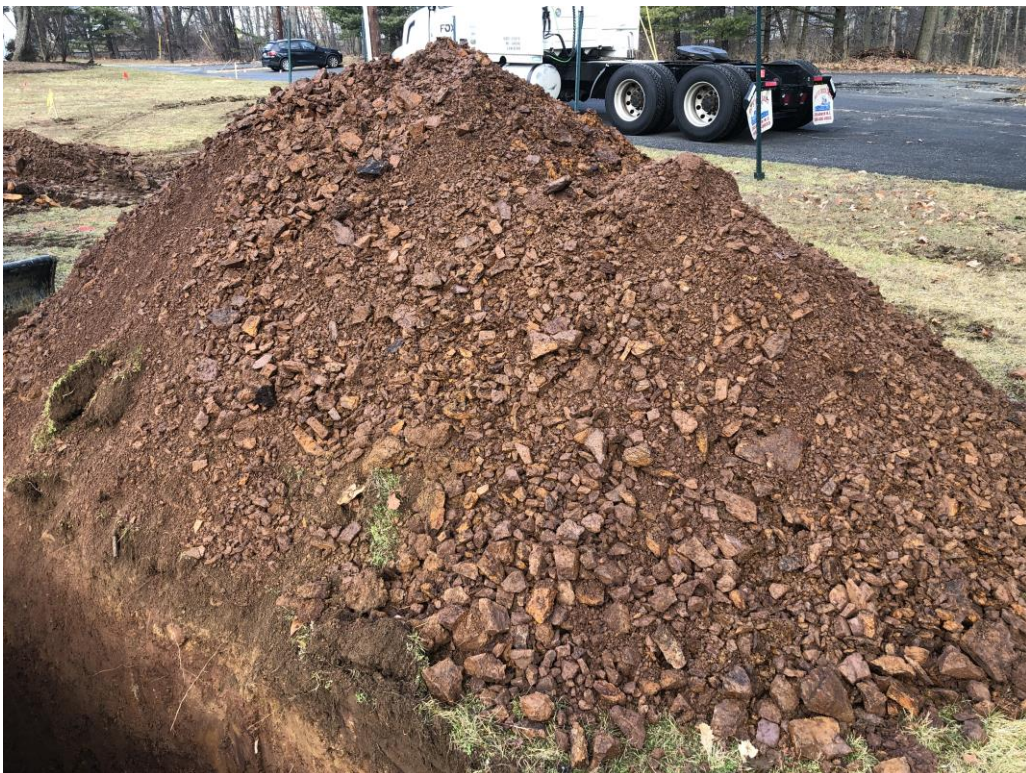
Photo 29: Excavated material from Test Pit STP-10.
