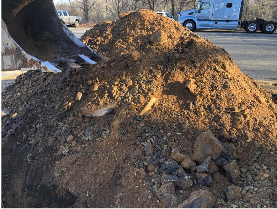
Photo 32: Excavated material from Test Pit STP-11.
