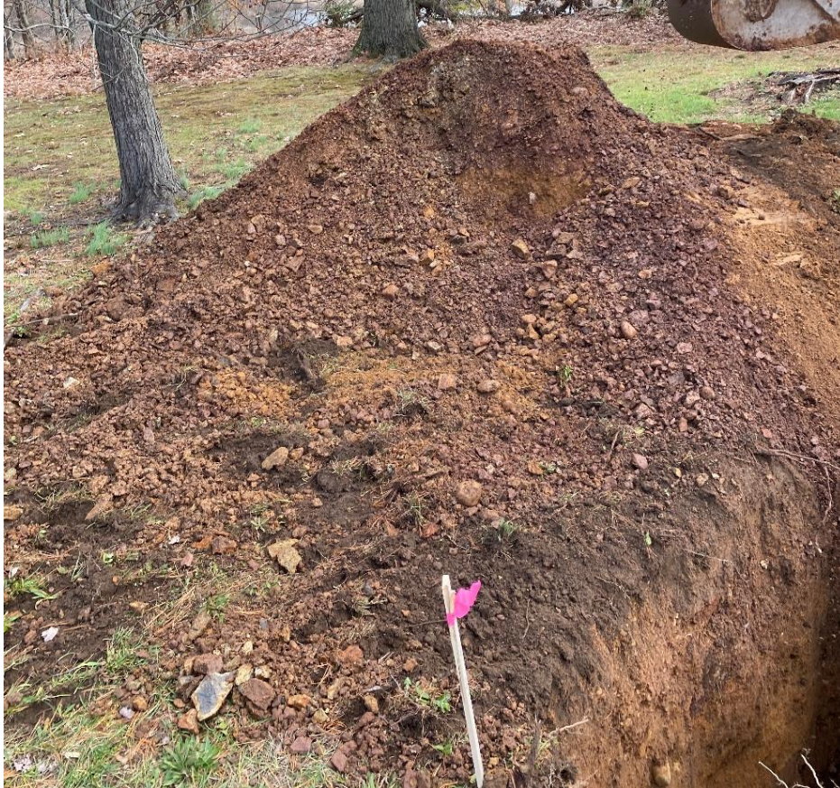
Photo 14: Excavated material from Test Pit TP-1.
