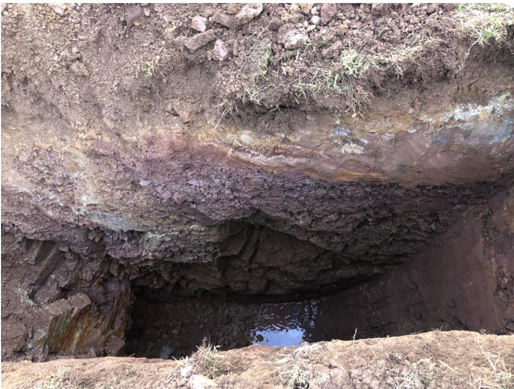
Photo 25: Profile of Test Pit STP-9.
