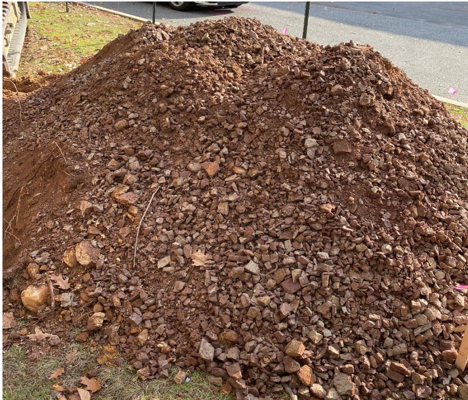
Photo 23: Excavated material from Test Pit TP-4.
