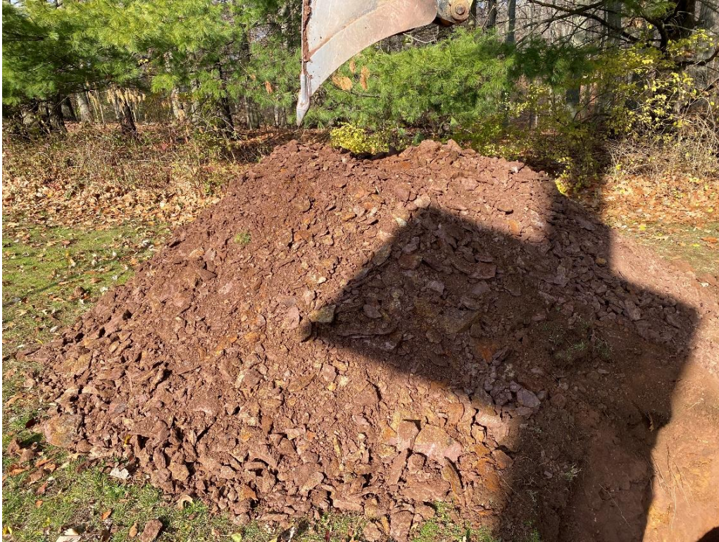
Photo 20: Excavated material from Test Pit TP-3.
