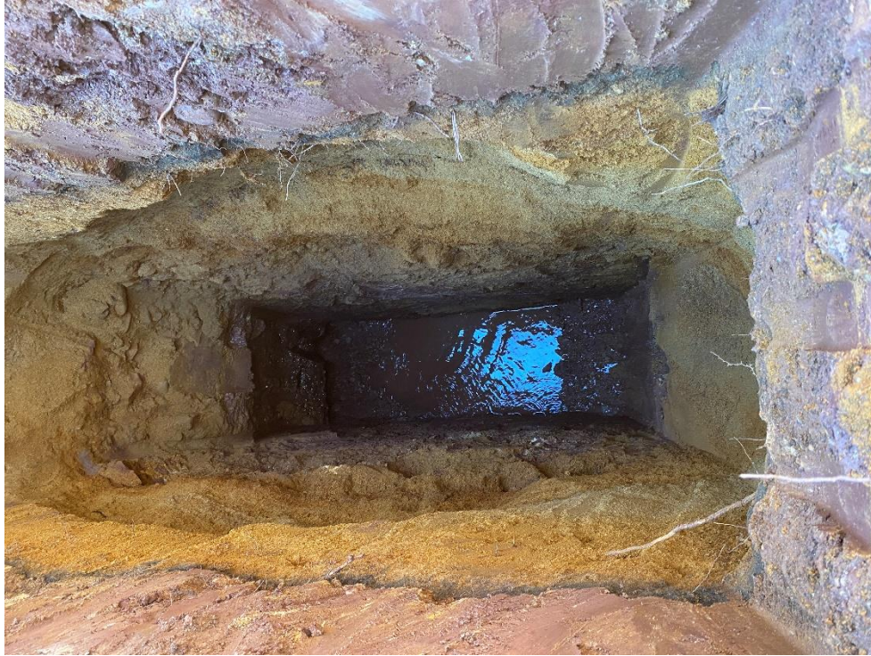
Photo 1: Profile of Test Pit SHGW-1.
