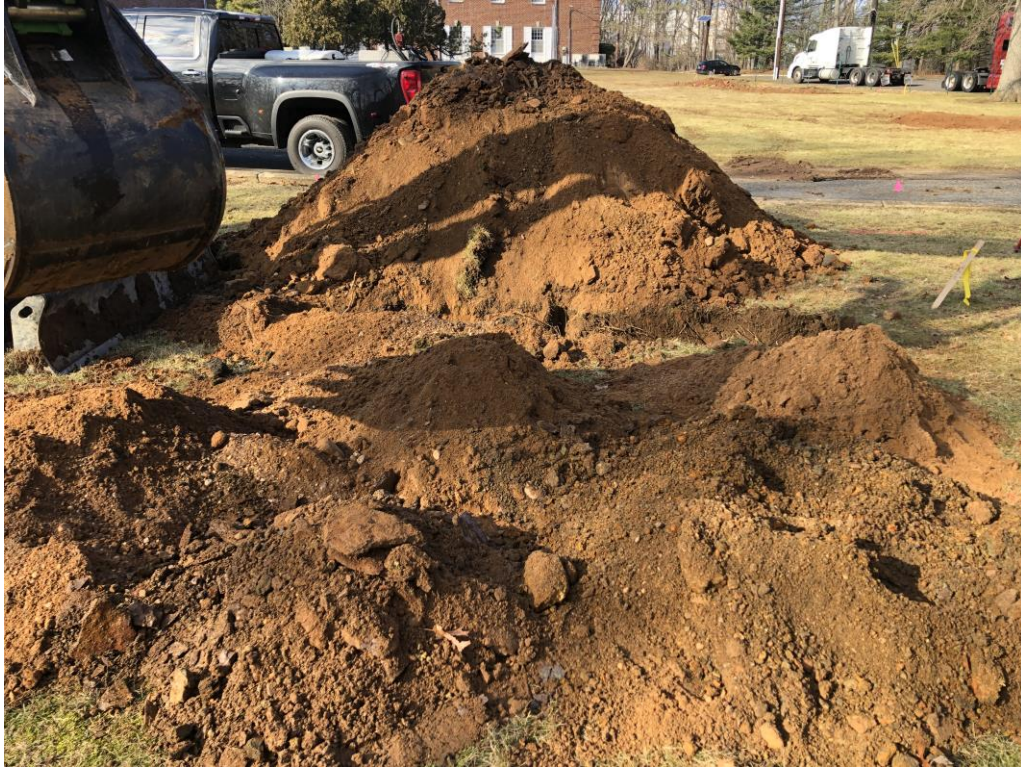
Photo 20: Excavated material from Test Pit STP-7.
