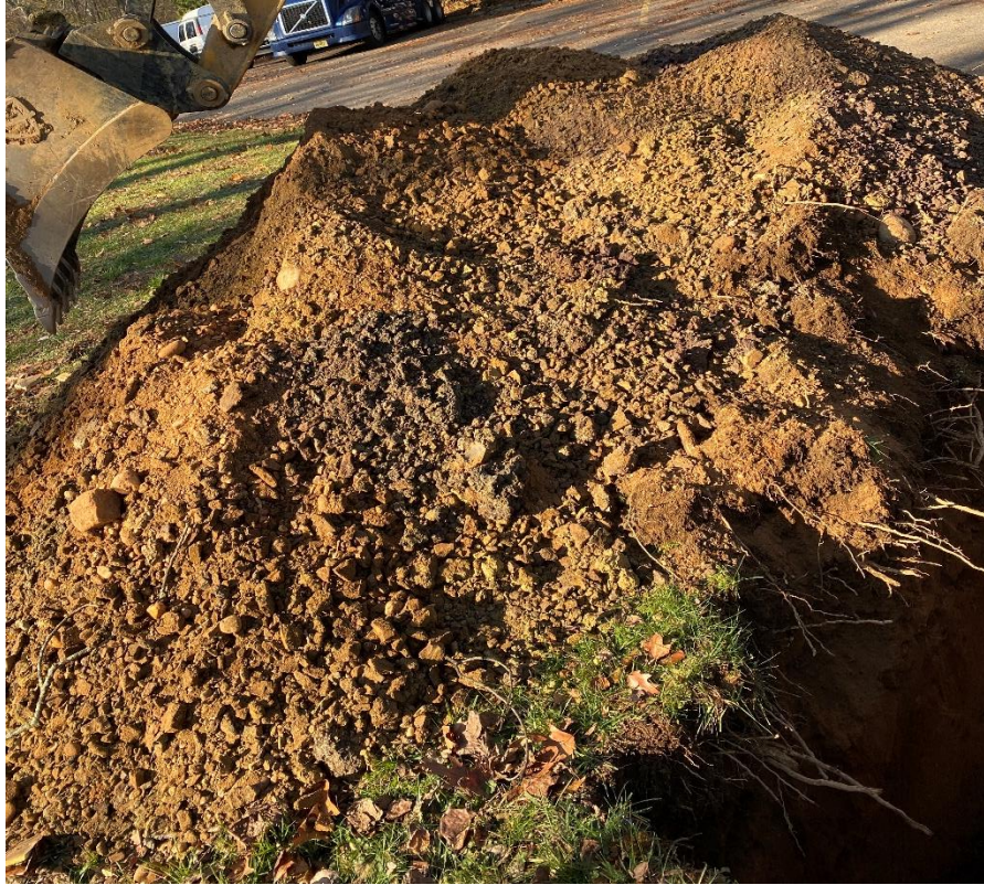
Photo 26: Excavated material from Test Pit TP-11.
