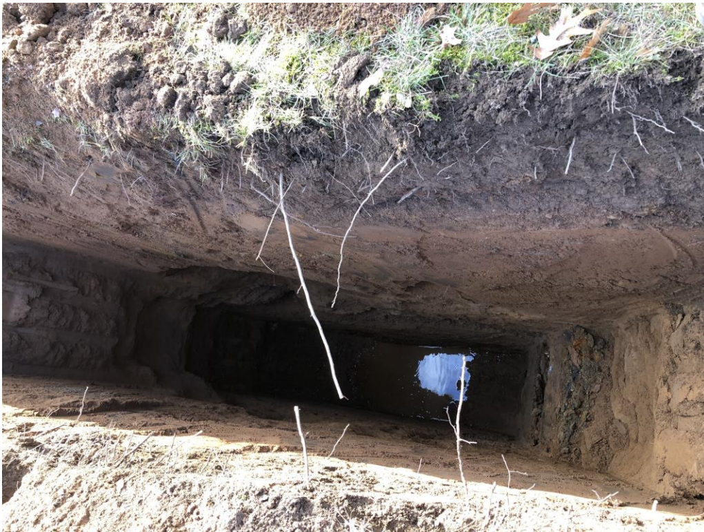
Photo 21: Different view of soil profile in Test Pit STP-7.
