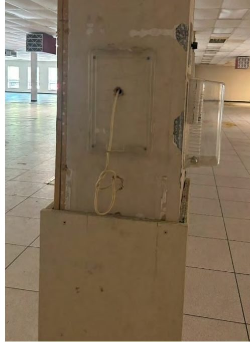
Figure 23 (Left) – Remains of an old air conditioning unit, plugged haphazardly into the ceiling. Figure 24 (Right) – Exposed wiring from an old thermometer.
