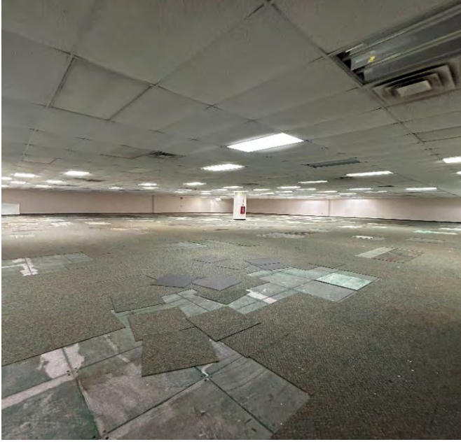
Figure 14 (Left) – Open concept floor plan of the old Data Center. Figure 15 (Right) – Damaged ceiling and floor tiles and loose wiring within Building 230.
