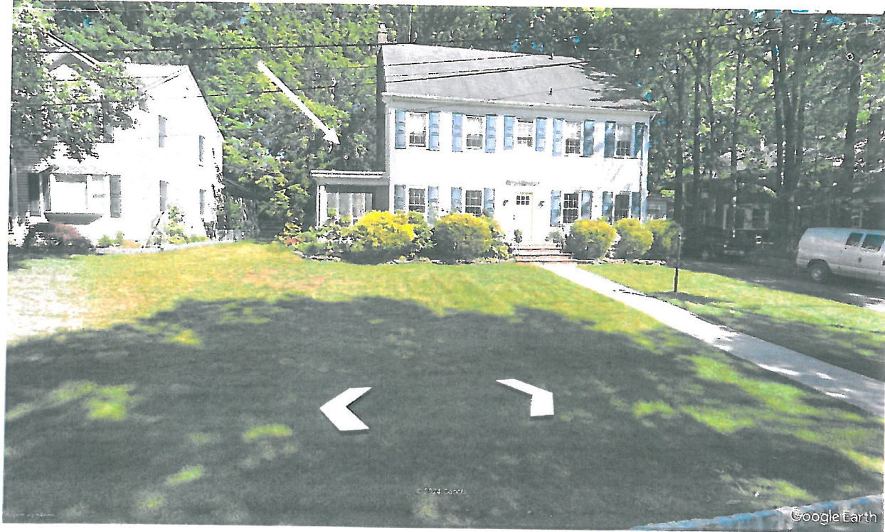
Area above sunroom where addition was constructed
