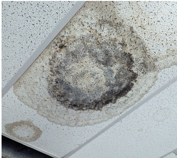
Figure 19 (Left)– Evidence of water damage within the ceiling tiles in Building 180. Figure 20 (Right) – Inactive light fixtures left abandoned.
