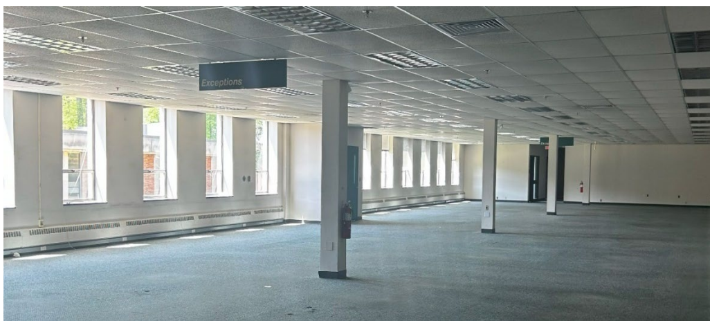
Figure 22 – Vacant office space, formerly an Exceptions Department for Wells Fargo.
