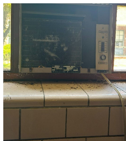
Figure 29 (Left) – Rusted and exposed wiring within the kitchen. Figure 30 (Middle)– Evidence of animal droppings within on the kitchen floor. Figure 31 (Right) – Evidence of animal droppings on a windowsill in a kitchen storage room.
