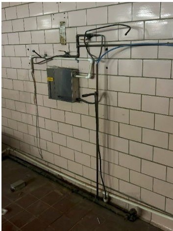
Figure 29 (Left) – Rusted and exposed wiring within the kitchen. Figure 30 (Middle)– Evidence of animal droppings within on the kitchen floor. Figure 31 (Right) – Evidence of animal droppings on a windowsill in a kitchen storage room.
