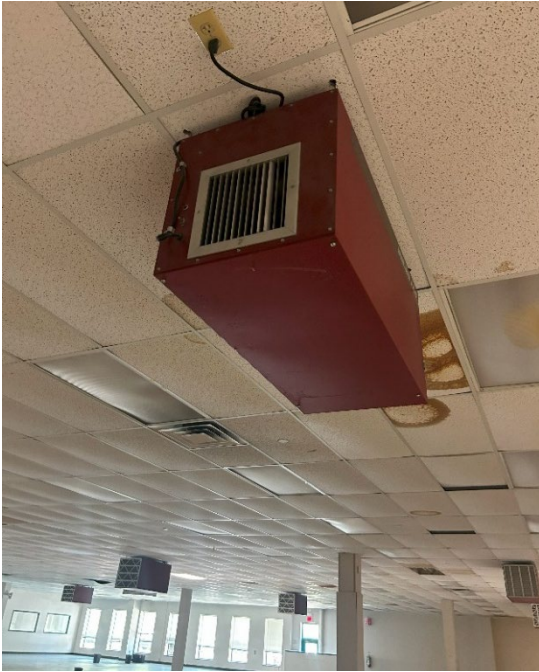
Figure 23 (Left) – Remains of an old air conditioning unit, plugged haphazardly into the ceiling. Figure 24 (Right) – Exposed wiring from an old thermometer.
