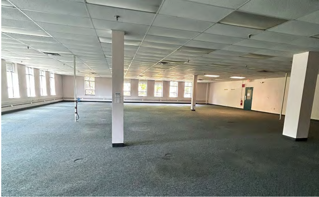
Figure 10 – Vacant office space within Building 100.
